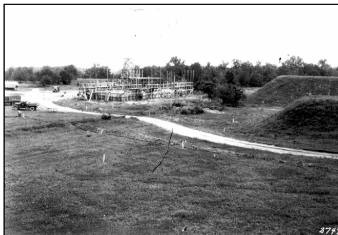
Figure 4.6. Photograph taken in August 1938 of museum construction. The photograph was taken looking north-northwest, from atop Mound N, and shows two mounds, Mound O the closest and Mound P in the distance. Note the fairly level ground and road running directly through where Lake #3 is located today. The original caption by Jones reads “Across lake and new museum looking northwest from Mound N. White stakes represent shore line” (courtesy of University of Alabama Museums, Tuscaloosa, Alabama).
